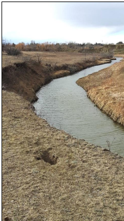
Picture 8 - Looking west at Pothole Creek within segment 8
