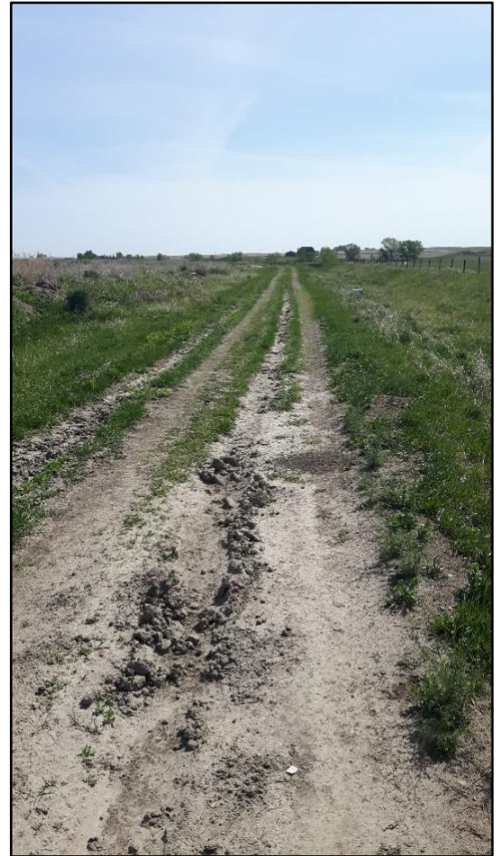
Picture 26 - Looking east, south of former sewage lagoons, at primitive road in segment 13A (note that gravel road extends from 4 th Street E to a point approx. 30 m east of the most easterly new Town industrial lot)
