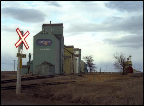
Magrath grain elevators (past & present) adjacent to former rail line
