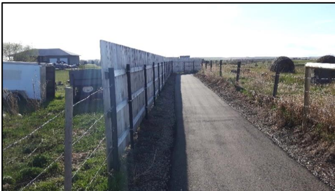
Looking west at fenced segment of outer loop
