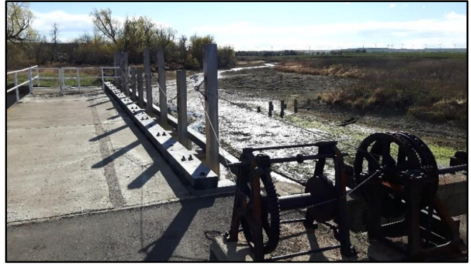
Looking southwest from the Magrath Irrigation Headworks
