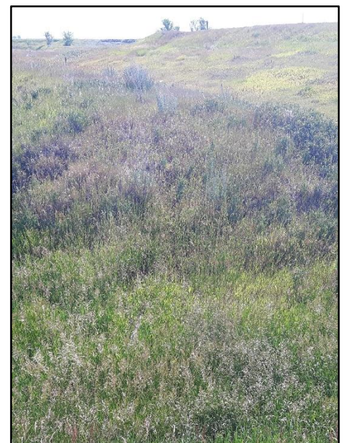
Picture 12 - Looking east at cut in irrigation bank (potential spot to get atop of irrigation canal bank) within segment 9
