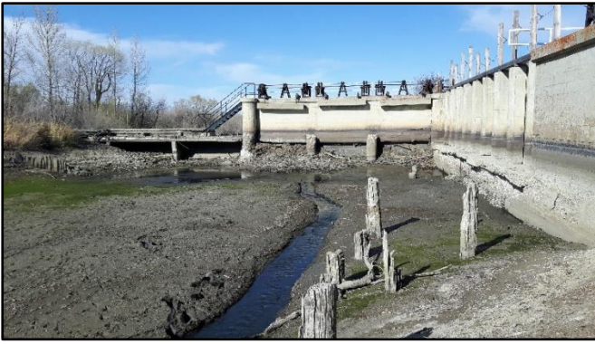
Upstream of the Magrath Irrigation Headworks looking northeast
