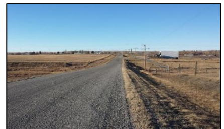
Looking west at 5 th Avenue S (being the Town/County southerly boundary) with the waste transfer station in the background
