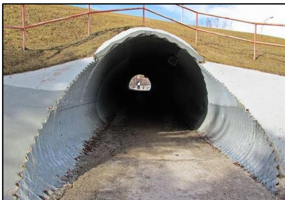
Walking trail tunnel beneath roadway in Confederation Park (Calgary, AB)
