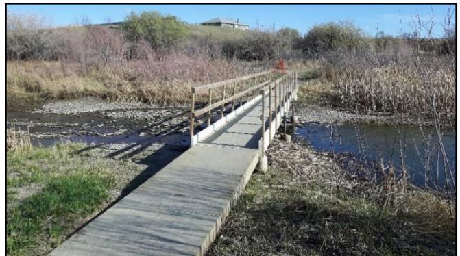
Looking south at temporary bridge over Pothole Creek (replaced in August 2016)
