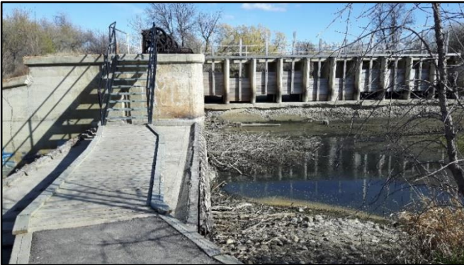
Looking south at pedestrian access over Magrath Irrigation Headworks
