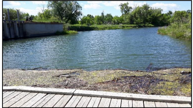
Looking west upstream of Magrath Irrigation Headworks
