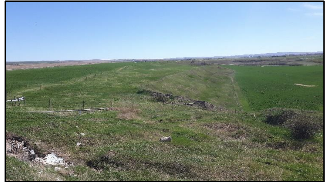
Picture 79 - Looking south at irrigation canal right-of-way from County road allowance
