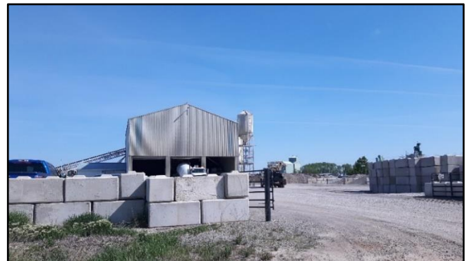
Picture 52 - Looking north from 2 nd Avenue N at Southwest Concrete, located to the south of segment 23
