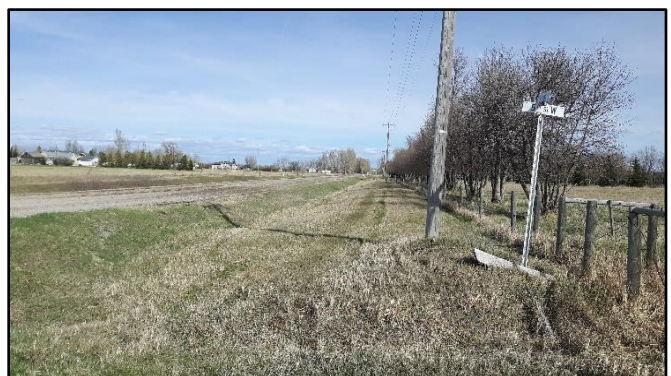
Picture 66 - Looking east at segment 25 within 5 th Avenue S right-of-way, adjacent to 5 th Street W
